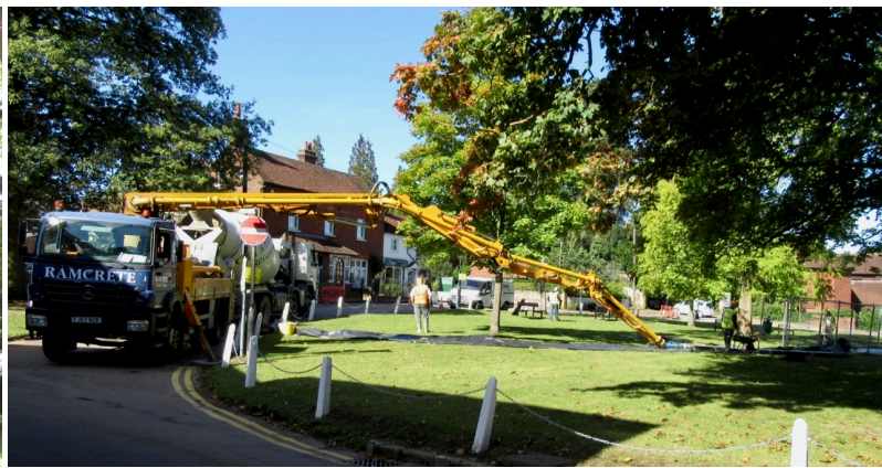
Pumping concrete into the shelters at Bowers Way (left) and Leyton Green (right).
